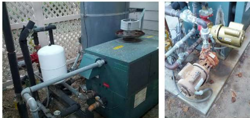
Figure 2 – Typical boiler, storage tank, and recirculation pump arrangement for a single Raydronics loop
