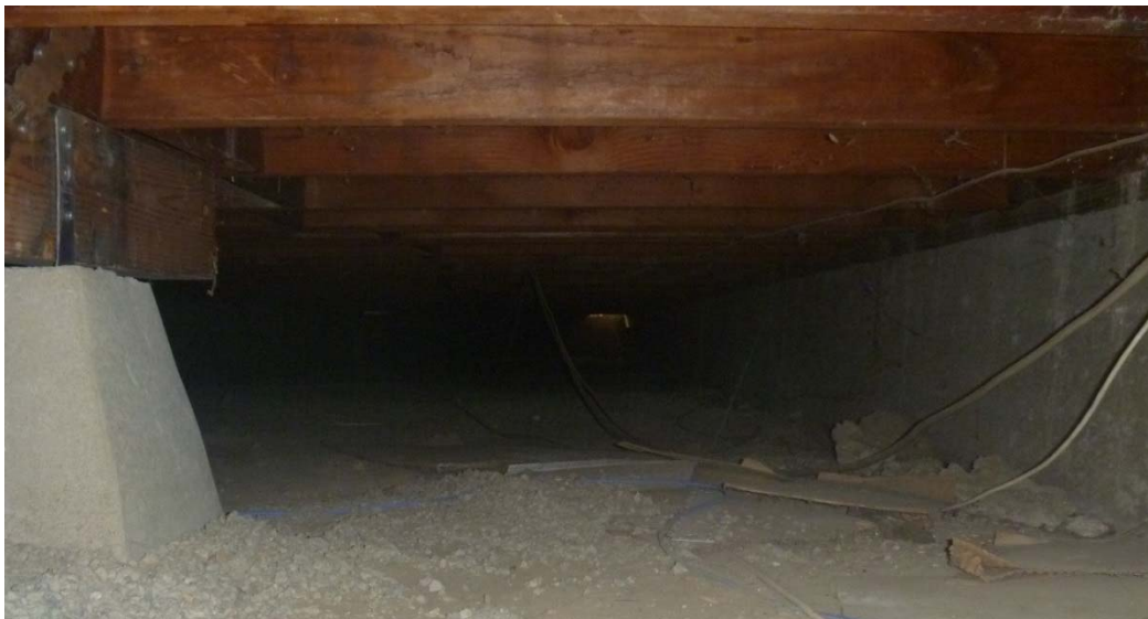
FIGURE 1 – UNCONDITIONED, VENTED CRAWL SPACE EXAMPLE
