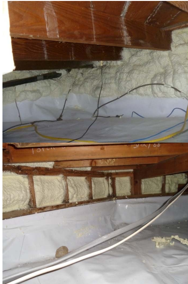
FIGURE 3 – VAPOR BARRIER AND INSULATION AFTER MEASURE IMPLEMENTATION
