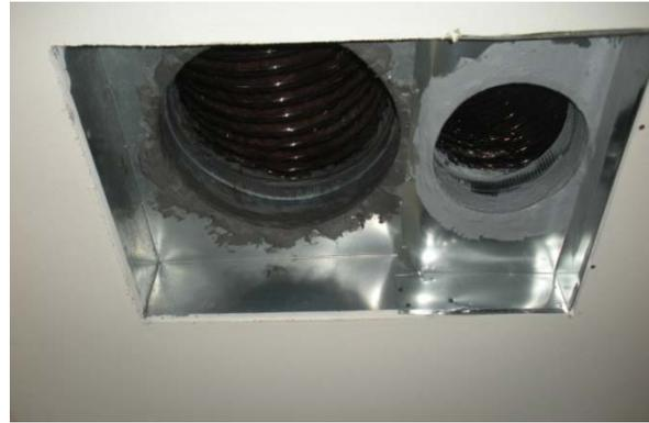
**Figure 30: System 4—New 10 in. to Plenum and 16 in. Into Blower Wheel Inlet Side With Metal Elbow**
