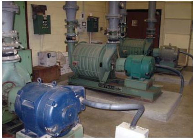
Figure 1: Hoffmann Blowers at Pana WWTP
